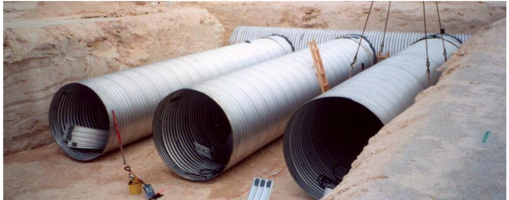
Aluminized Steel Type 2 was developed for superior environmental corrosion resistance.
